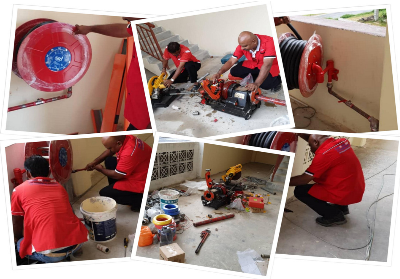
HOSE REEL INSTALLATION
