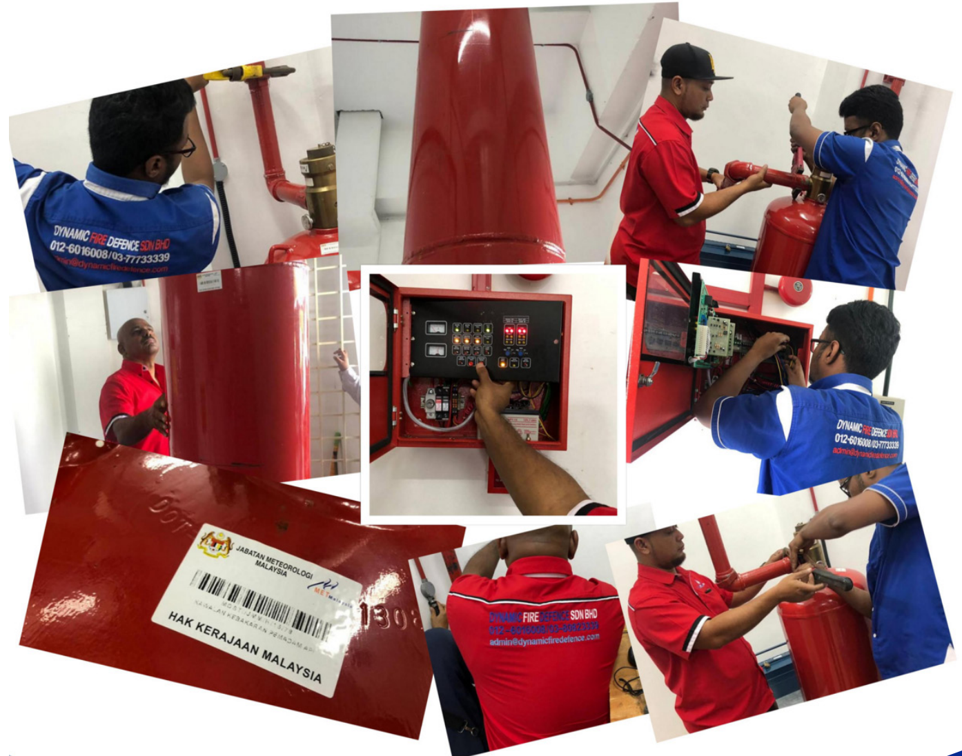
FM200 SYSTEM INSTALLATION
